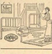
The slightly raised edge confines the mattress to the top of the spring and it cannot spread over the sides.
